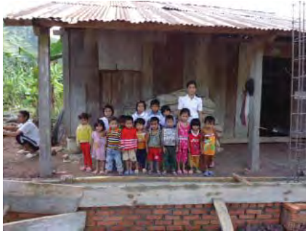
Ca Tu kindergarten children watching new kindergarten construction
